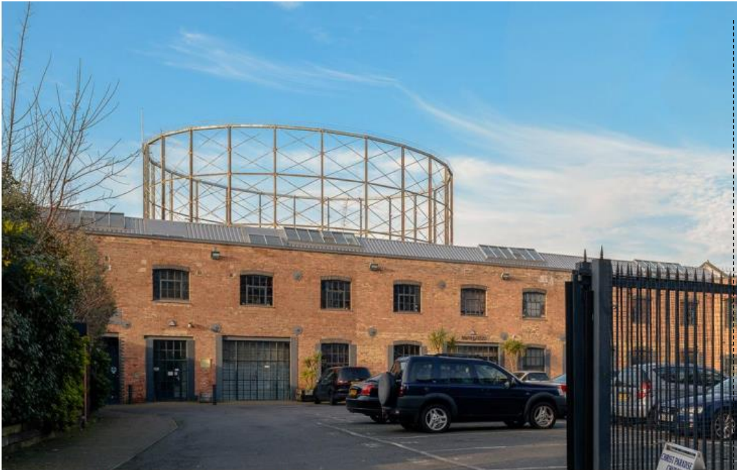
Existing converted 1920's warehouse building, housing a business park.
